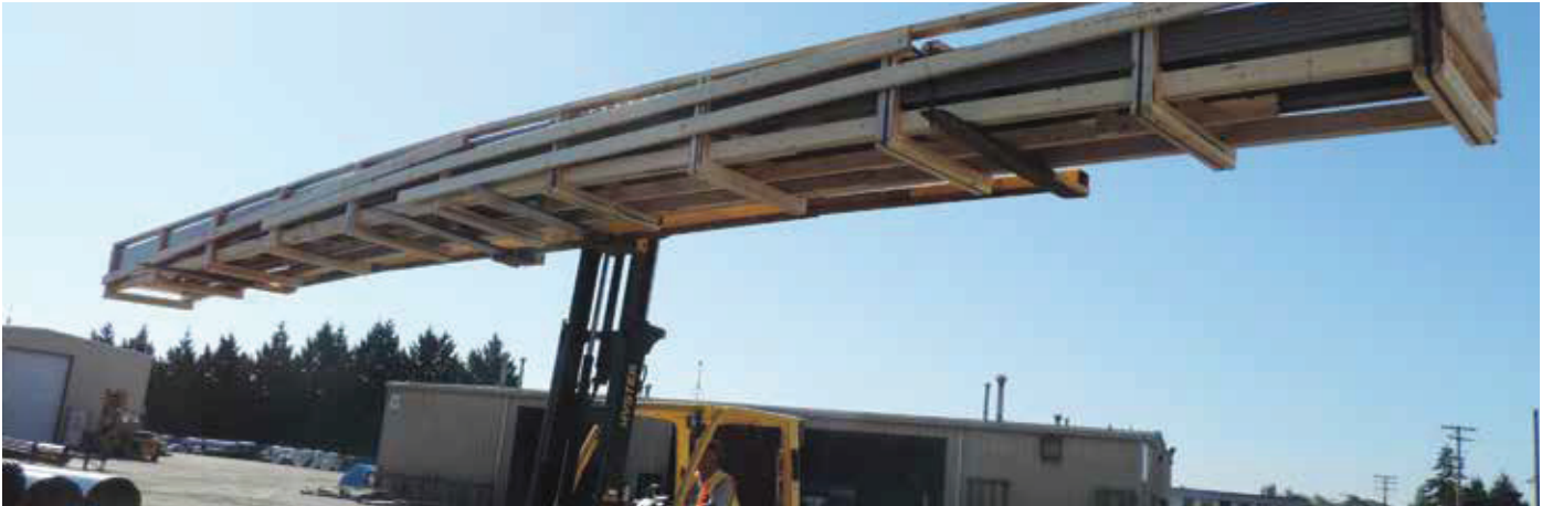
Use spreader bar with a forklift.
