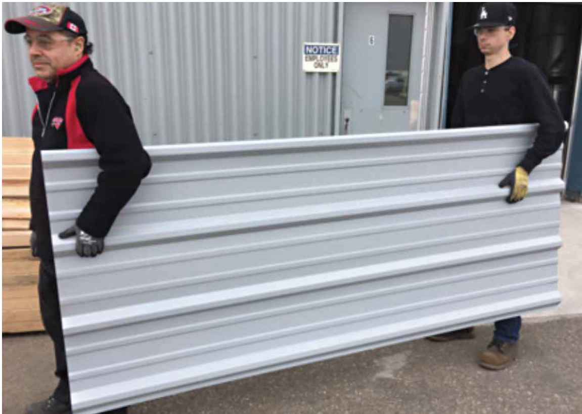
The correct way to carry a profiles sheet
