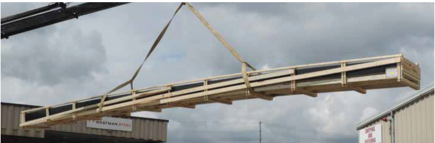
Using a nylon strap when utilizing a crane for lifting.
