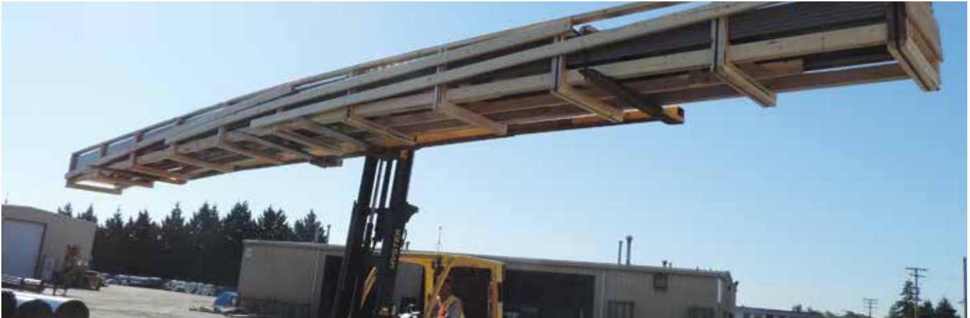
Use spreader bar with a forklift.
